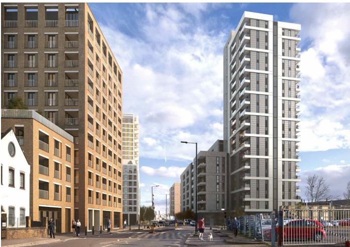
North Kensington Gate on left, proposed Mitre Yard scheme on right, looking south on Scrubs Lane
