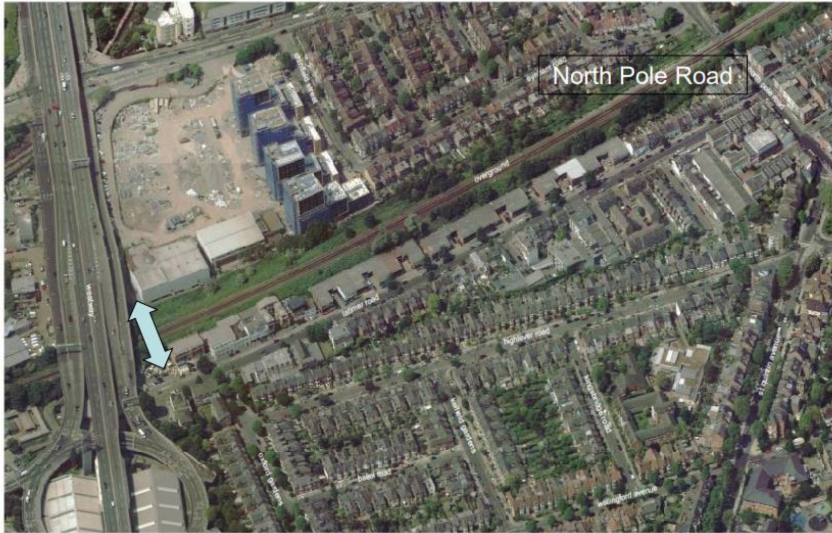
Aerial view of suggested site for WLL station at Westway roundabout, showing location of planned pedestrian/cycle underpass between Imperial West and Latimer Road
