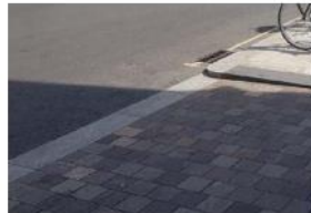
Parking bays paved with Porphyry setts
