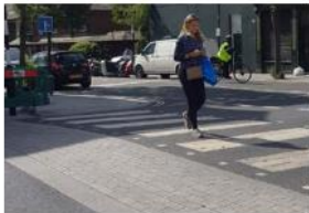
Raised tables with granite ramps
