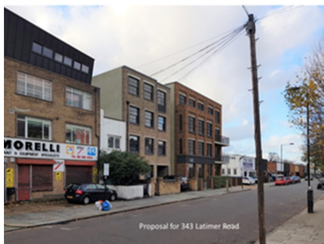
The Morelli building, Nos 341A and 341, and redeveloped Unit 1
